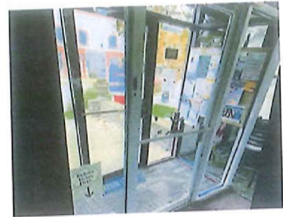
These doors included (interior sides only)
