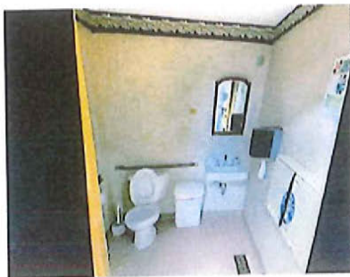
Pull wall paper and paint this bathroom
