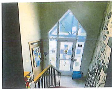
No brick to get painted
